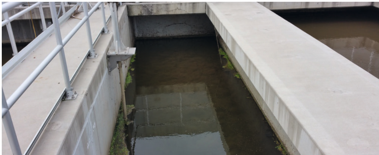
Before the Landia mixers were installed at Milton, where the greenery at the edges shows that the tanks needed proper mixing
